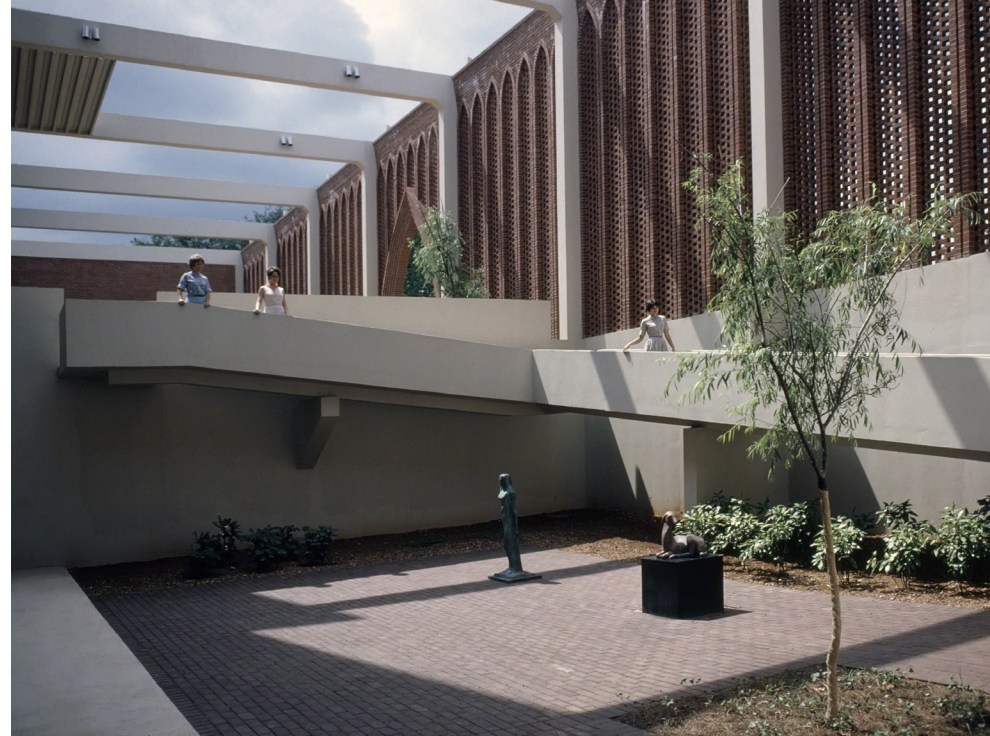
A cantilevered ramp leads from the ceramics area at ground level out to a sculpture court.
