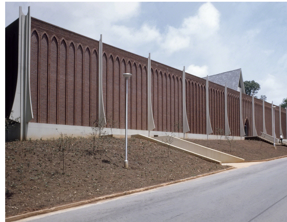
A rear view shows the great corbeled brick wall and exits leading to Dougherty Street.
